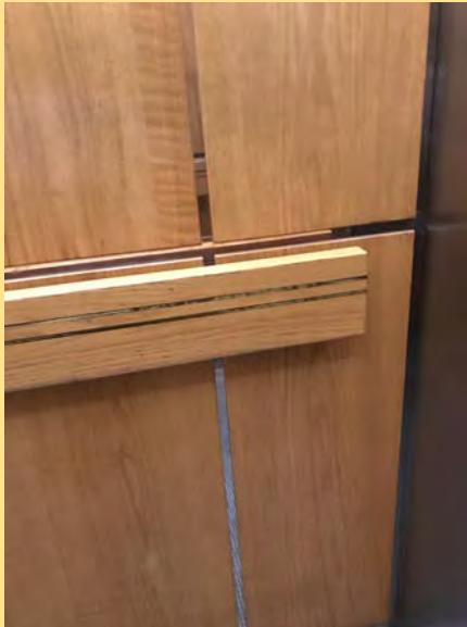
Mirror stainless-steel reveal that can be seen between wooden decoration panels
