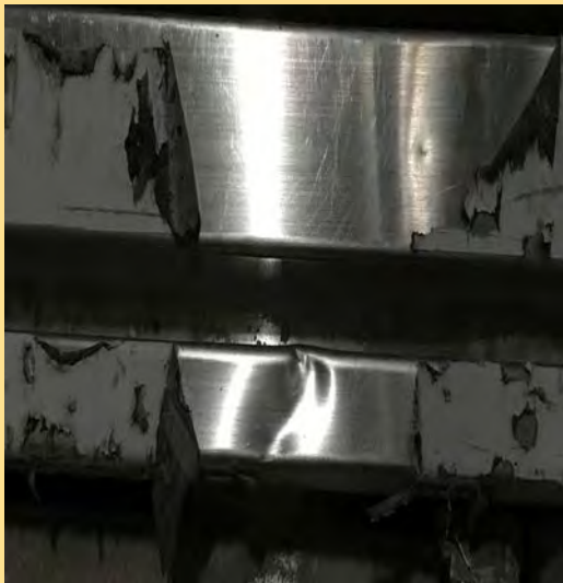
Damaged door sill with stainless-steel cladding
