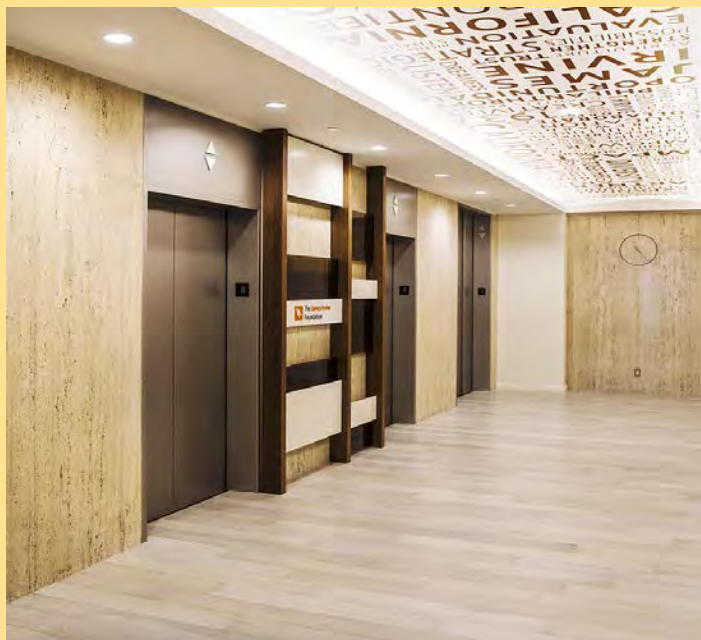
Hall lanterns mounted directly on the transom panel without a faceplate; source: ASD/SKY
