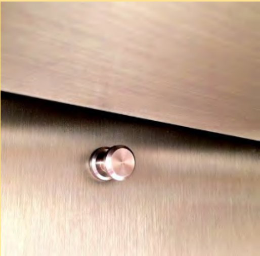
Permanent hook installed on car panel for suspending protective drapes; source: Kapok88
