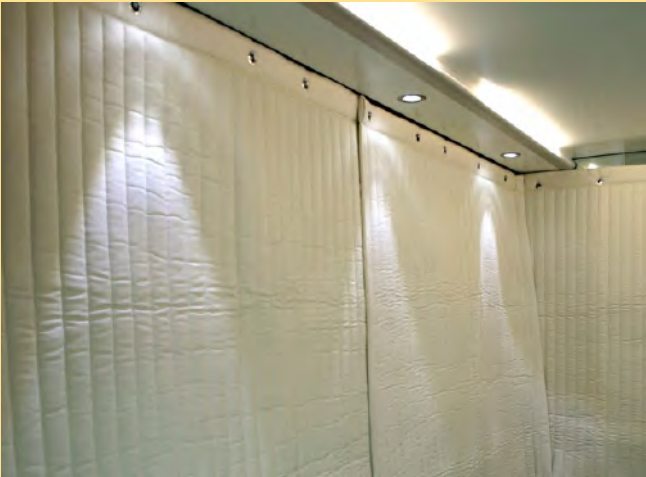
Protective drapes to protect car interior decoration; source: Kapok88
