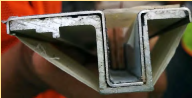
Aluminum door sill clad with stainless-steel sheet
