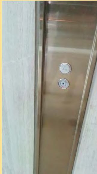
Hall call station, mounted directly on lobby wall without a faceplate
