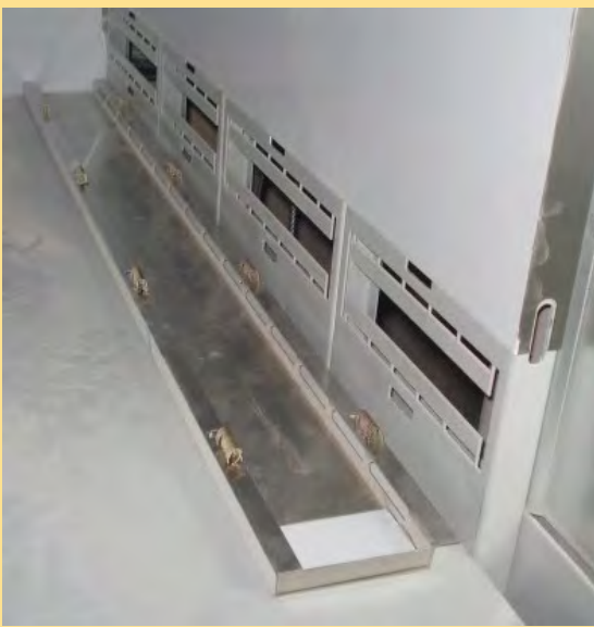
Ventilation slots hidden within the kickplate
